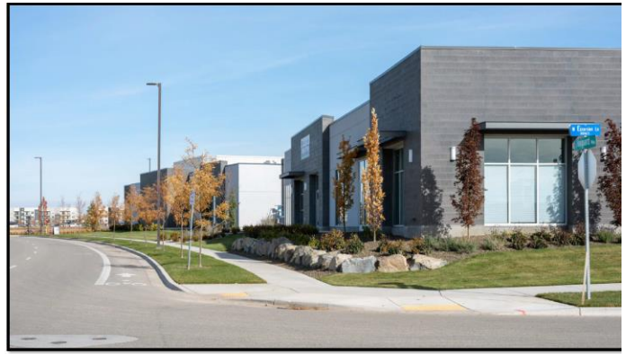
EXISTING SINGLE-STORY SHOPS
