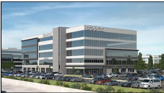
LASALLE BUILDING (under constr)
