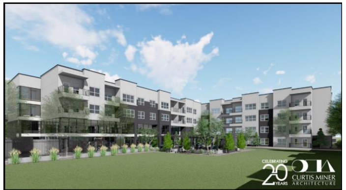
THE FLATS at TEN MILE (under constr)
