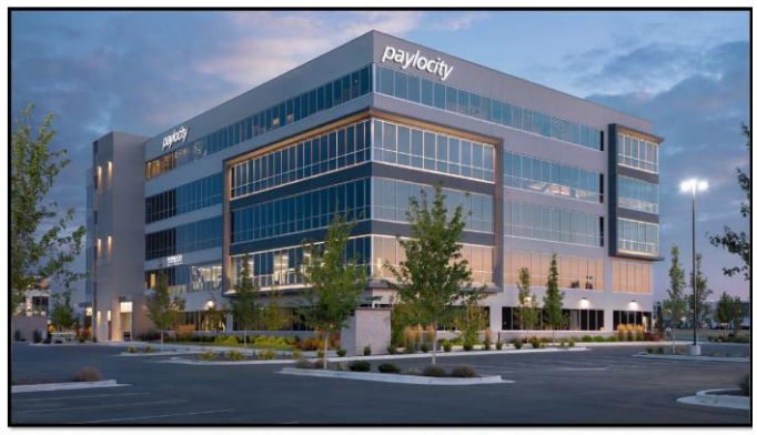
PAYLOCITY BUILDING (complete)
