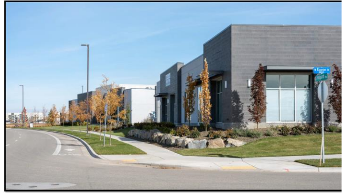
EXISTING SINGLE-STORY SHOPS
