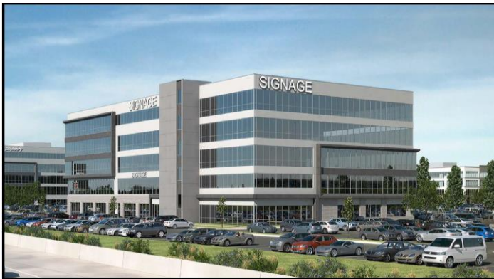
LASALLE BUILDING (under constr)
