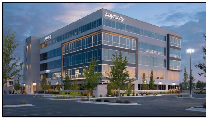
PAYLOCITY BUILDING (complete)
